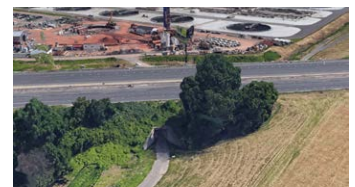
Connection under Levee
